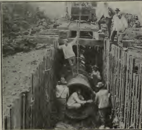
TYPICAL PIPE-LAYING CONDITIONS IN NEW ORLEANS
